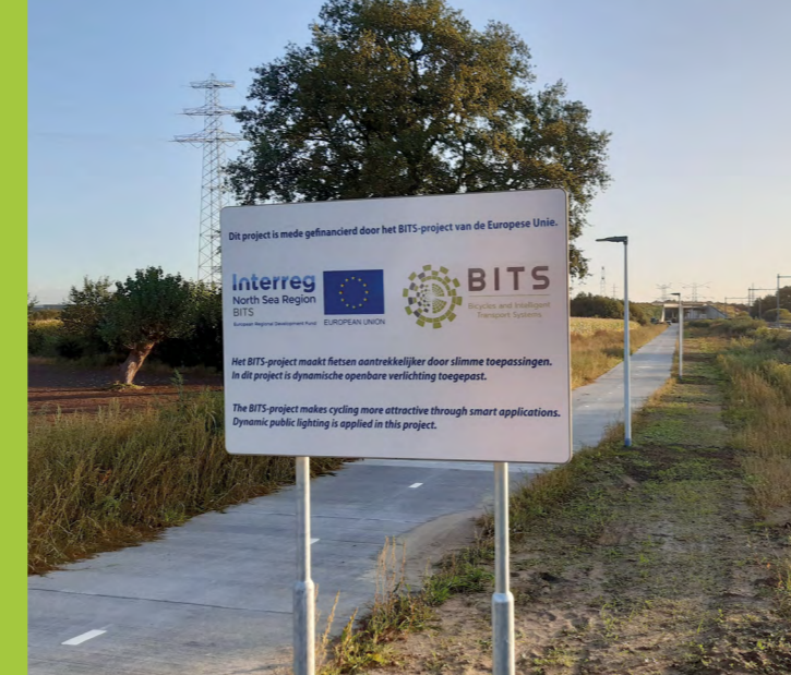
Figure 2.3: Dynamic lighting in Zwolle
